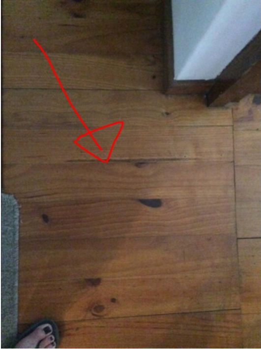
Lifting of floor boards
