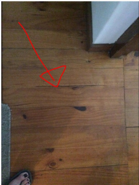
Lifting of floor boards
