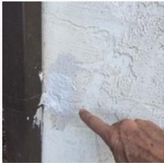
The back down spout hole has been repaired. Additional material will need to be applied.
