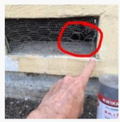
The 2nd crawl space vent has a fine mesh that has been damaged. Remove and replace.
