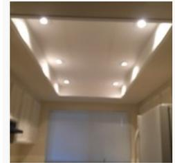
The corner edges will not be taped and textured, instead we are going to use a similar trim to those on the cabinet at the horizontal and vertical surfaces to cover wall board joints.
