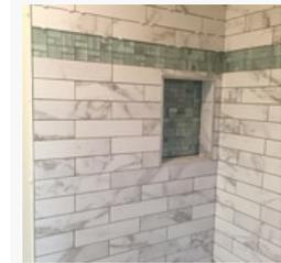
Shower: waterproof walls installed and nailed to studs. Water barrier added and final galvanized steel affixed.
