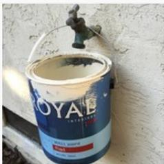
The tap has a constant leak and needs to be replaced.
