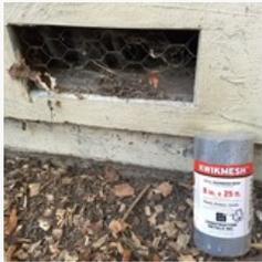
1 crawl space vent has no fine wire mesh and will need to be installed to control rodent access.
