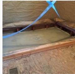
Wall: galvanized wire stapled up until neoprene liner is installed.
