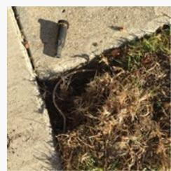
Repair broken sprinkler at driveway to walkway entry.
