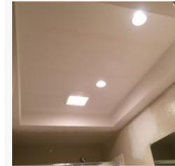
The original fan mounted in the wall has been removed. The hole has been filled and has been textured and is now drying.
