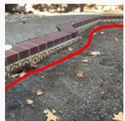
The fill has compacted and now the tile at prior water line is showing. Fill with dirt.
