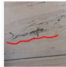
concern for wood borer – call fumigator 03/10/2015 11:15 (CAT)
