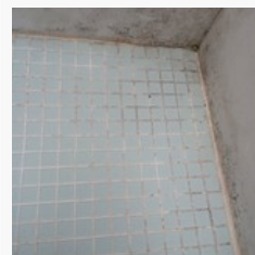
Mould present in shower to lower level 03/10/2015 11:25 (CAT)
