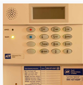
Alarm system 01/02/2017 15:07 (GMT)
