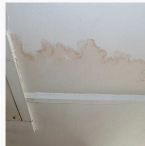
Bathroom ceiling stain 01/02/2017 15:07 (GMT)
