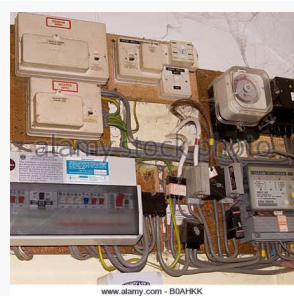
Electricity meter and fuse boxes 01/02/2017 15:07 (GMT)
